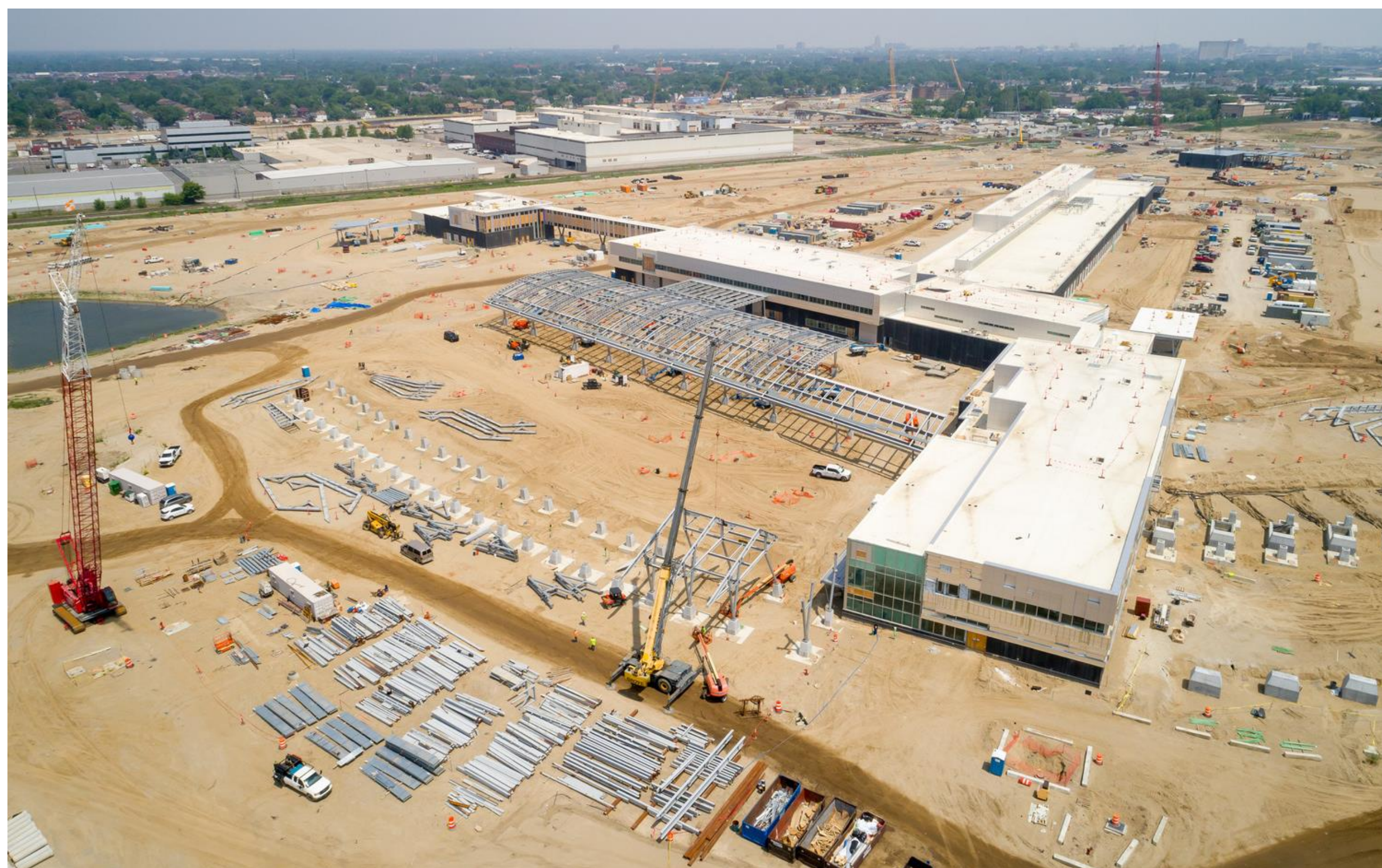
US Port of Entry construction progress
