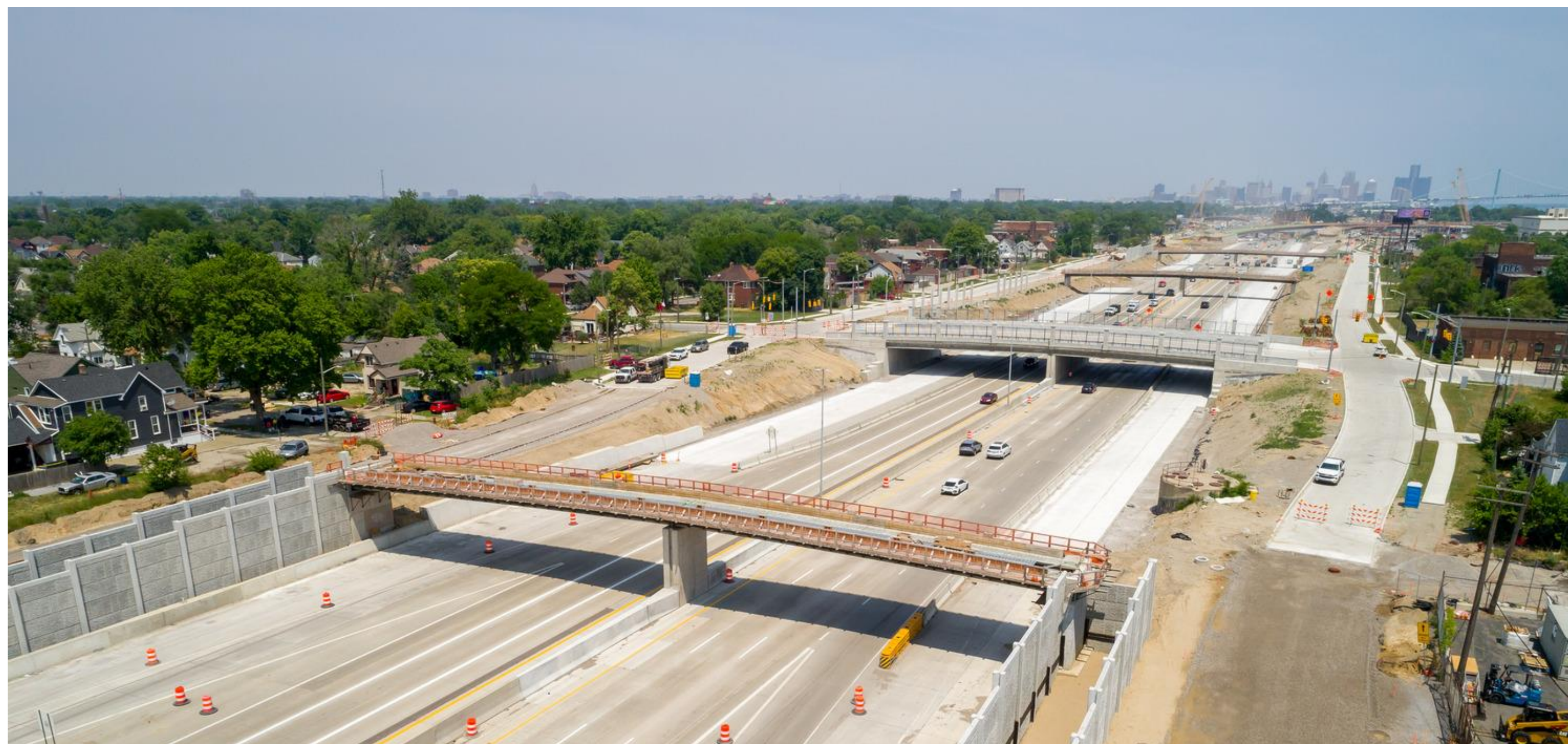
Solvay Street pedestrian bridge construction progress
