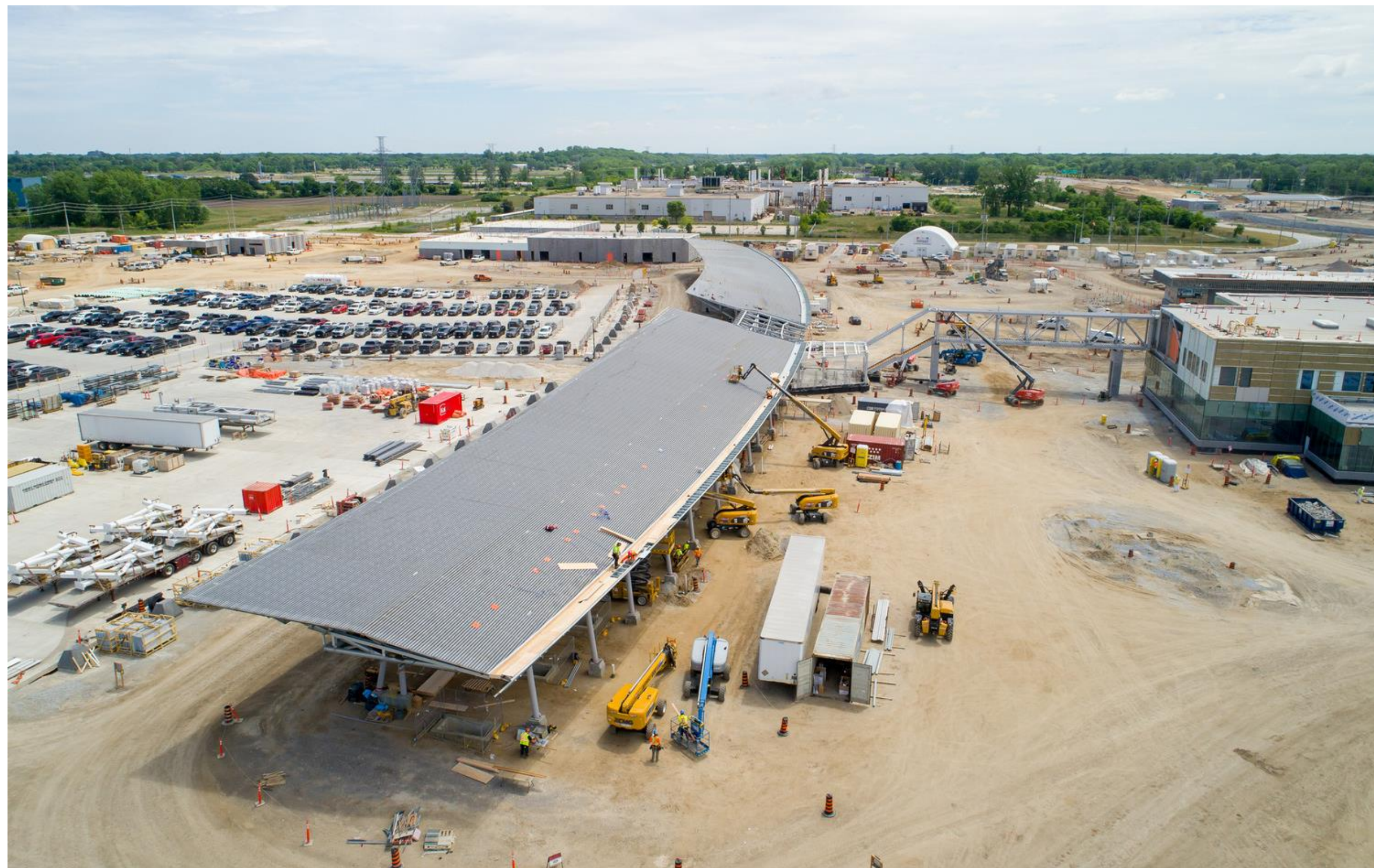
Canadian Port of Entry primary inspection lane canopy construction
