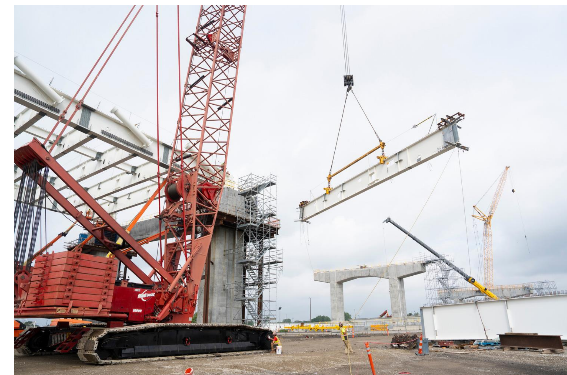
US bridge site construction progress (left photo) and road deck girder installation (right photo)
