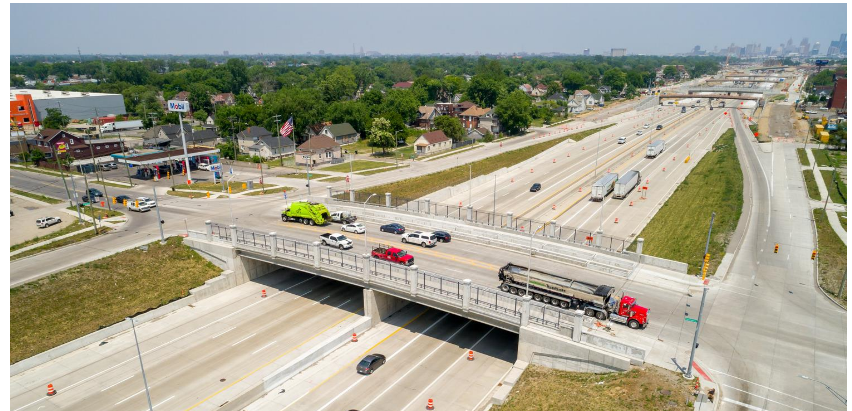
Springwells Street road bridge
