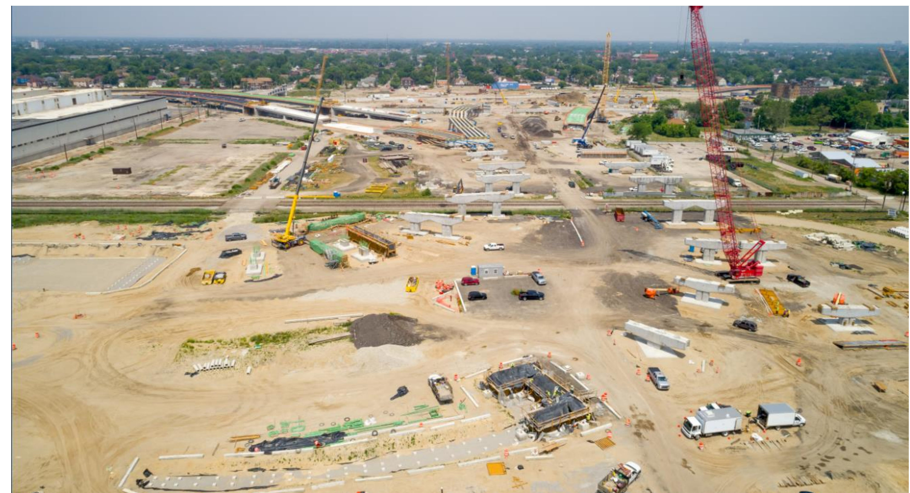
US Port of Entry construction progress
