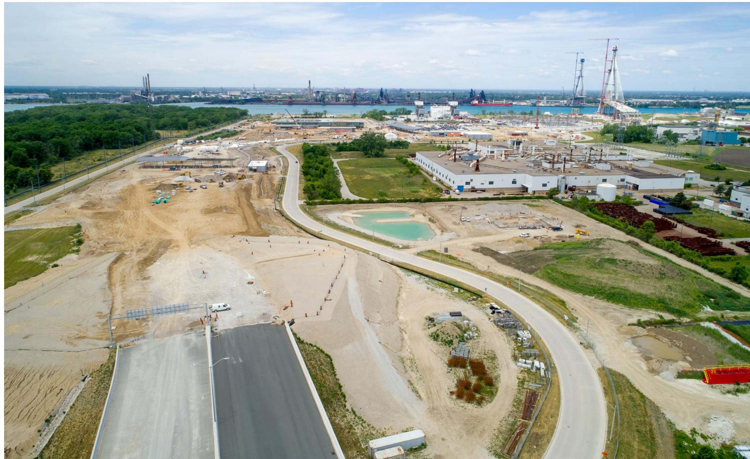
Canadian Port of Entry construction progress
