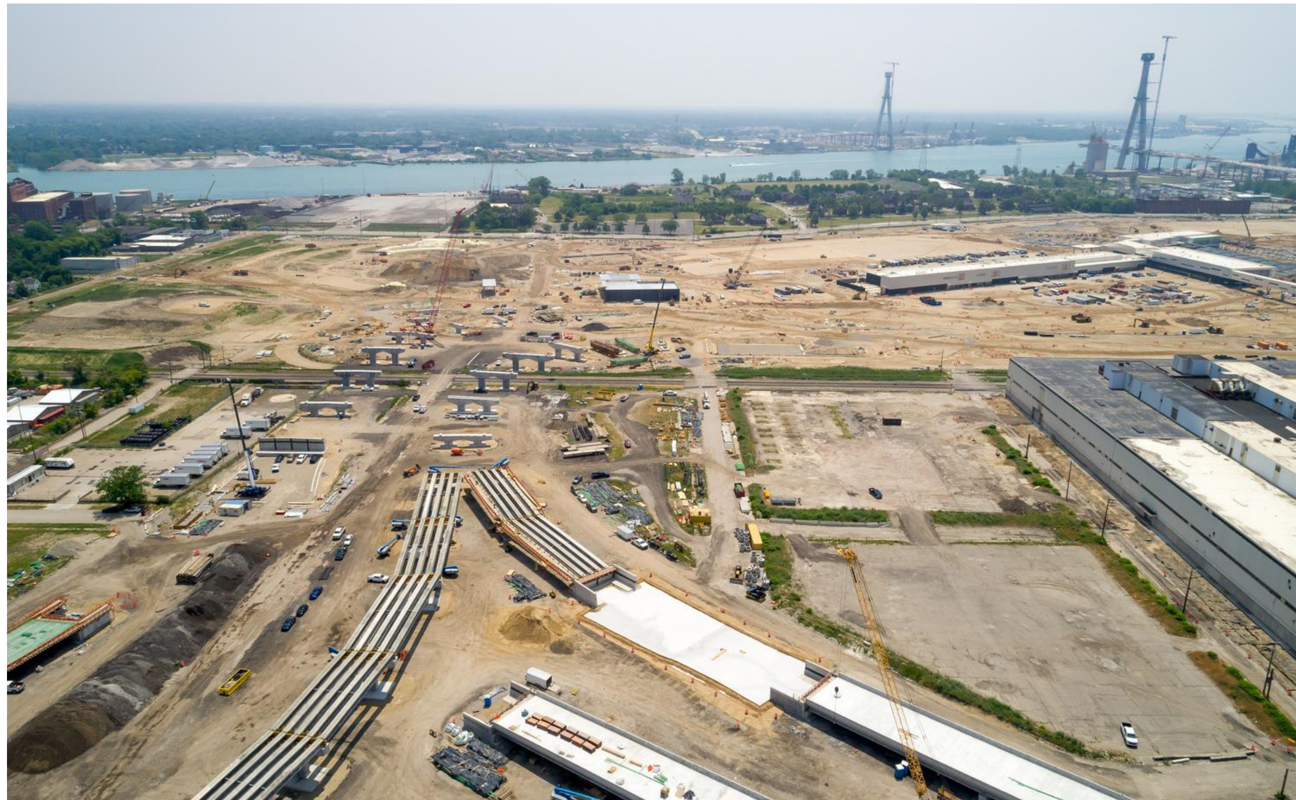
US Port of Entry construction progress
