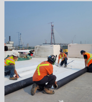
Quinn Roofing Solutions employees on the Canadian POE site.
