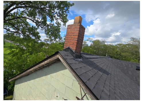
A completed roof repair through the Delray Home Improvement Program.
