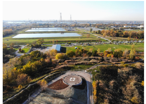
Aerial view of the Malden Park Observation Area during construction. A photo of the completed amenity is featured on the report cover.
