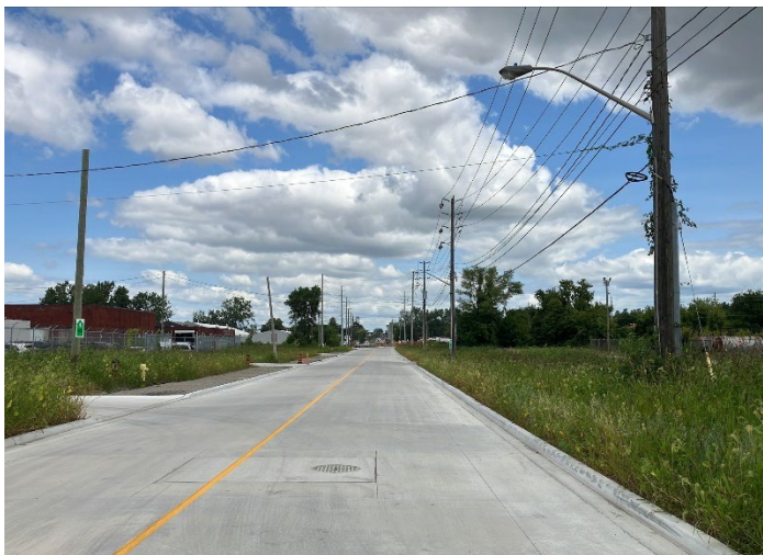
Sandwich Street Phase One reconstruction.
