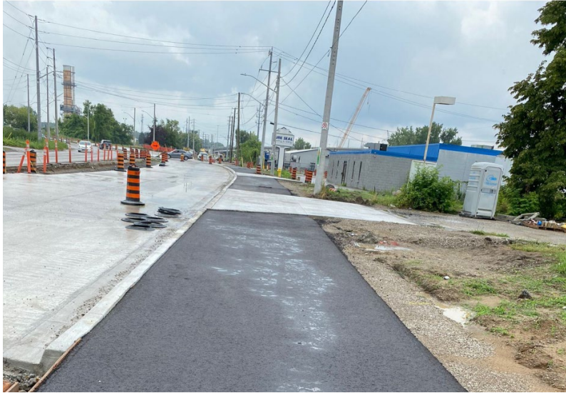
Above: Sandwich Street Phase Two reconstruction.
