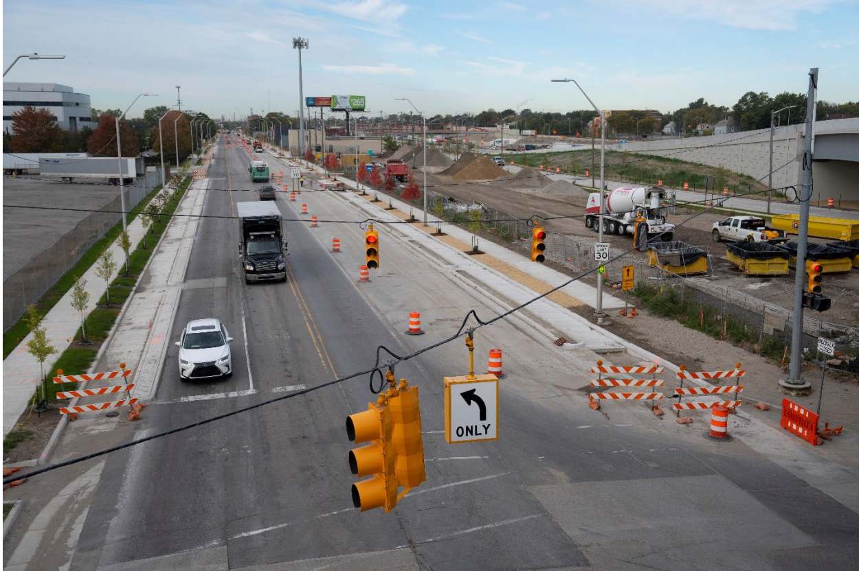
Fort Street local road improvement work.
