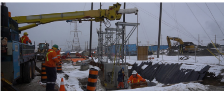
Hydro One transmission line work, Canadian Port of Entry
