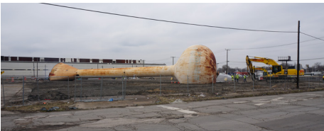
Water tower demolition, US Port of Entry
