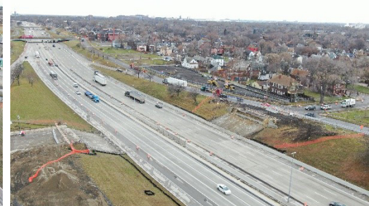
Post-demolition at Livernois Avenue bridge
