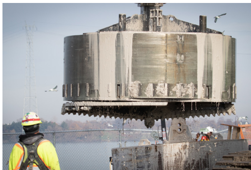
Prepping for drilled shaft installation
