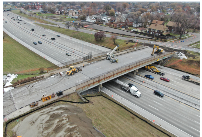
Pre-demolition at Livernois Avenue bridge
