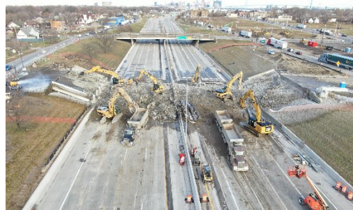
The Livernois Avenue bridge under demolition
